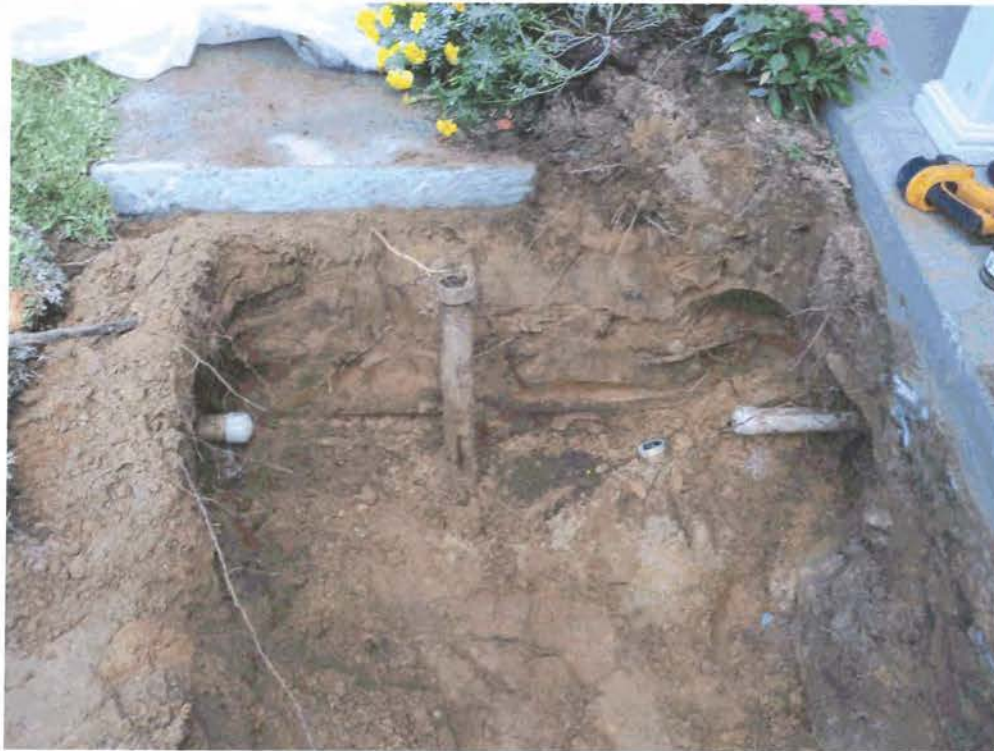
Picture 2: UST 151LaurelBB excavation in progress.
